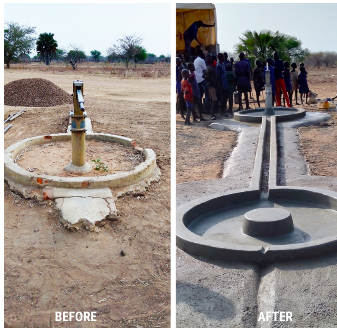
Rehabilitated well at Panmil primary school
